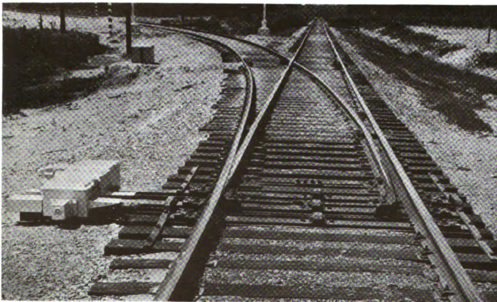
View of the new junction switch showing electric machine and the special plates and rail braces
