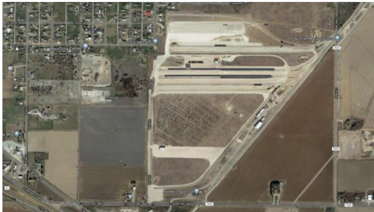
South Plains & Lamesa Railroad – Rail port facility at Slaton, Texas
